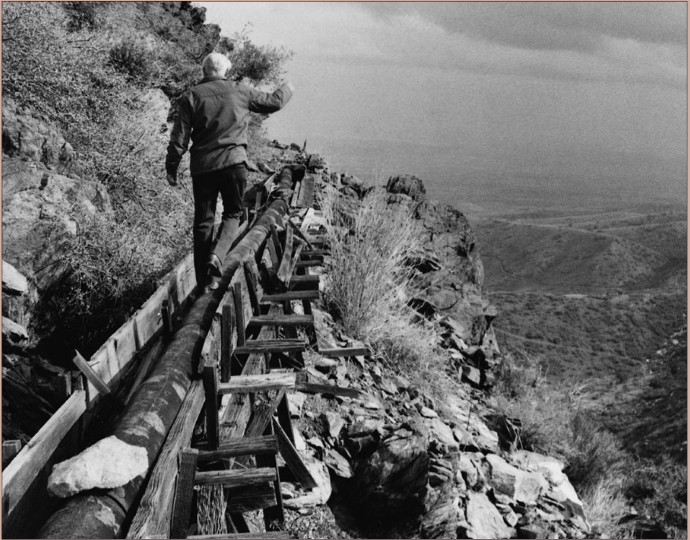
Stewart Young of Kerona, Inc., walks a precarious path — the water supply line for Jerome, Arizona, that ends in Deception Gulch.
