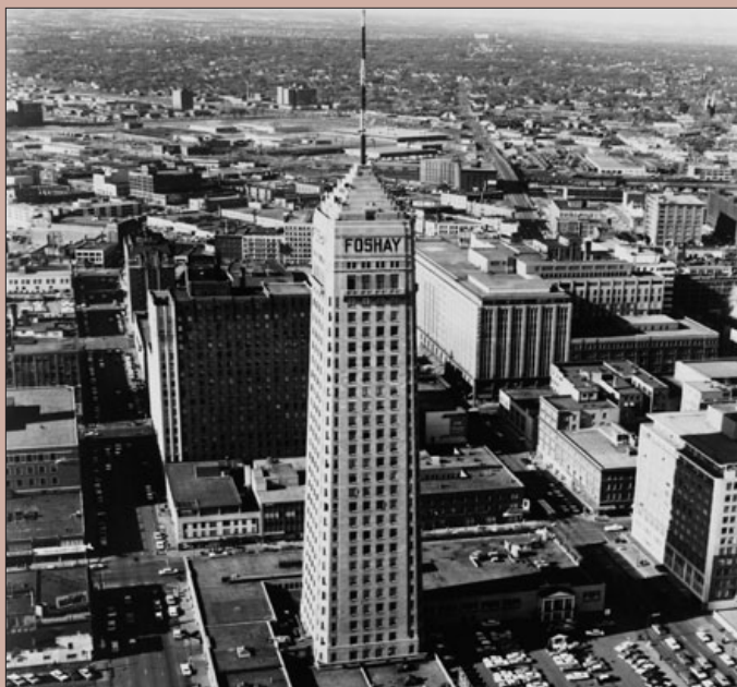
The Foshay Tower, which for nearly half a century was the dominant feature of the Minneapolis skyline, served as Apache’s corporate headquarters until late 1984.
