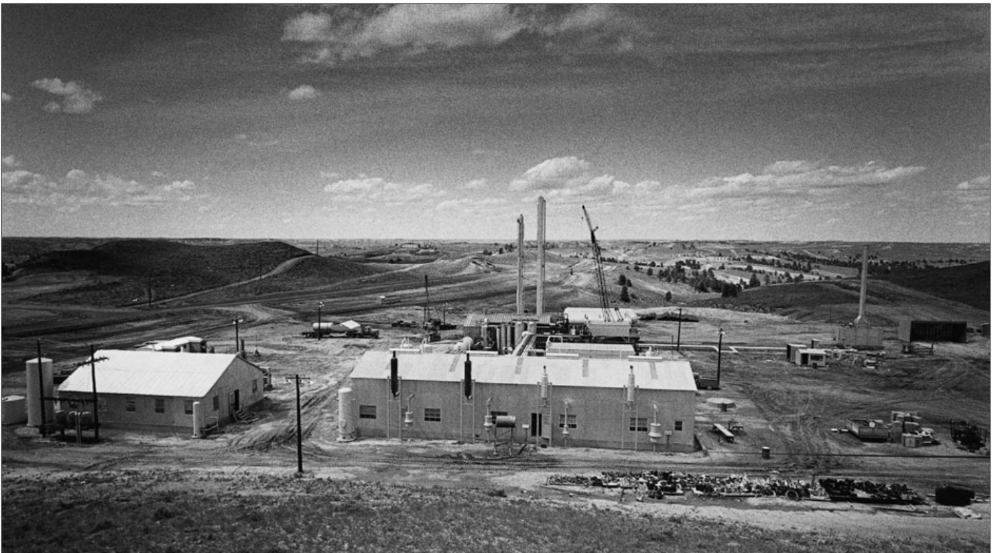
Apache's gas plant at Recluse
