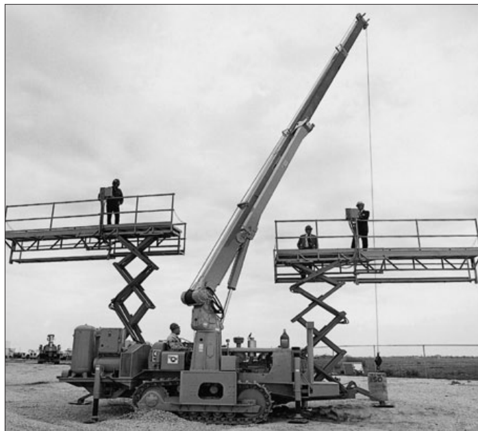
Apache's National Crane subsidiary designed and manufactured this special equipment for use in building the Alaskan pipeline. The design allowed equipment to work without sinking into and damaging the fragile permafrost terrain.
