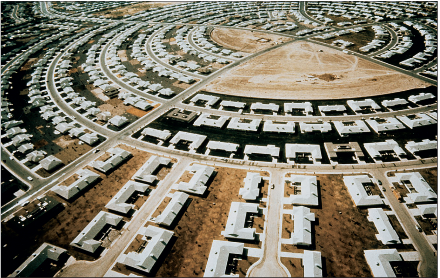
The fast growth of Goettl Bros. Metal Products, a leading manufacturer of climate control systems for the Southwest, coincided with the population explosion in the Sun Belt states. Large developments like this Sun City retirement community in Arizona featured Goettl air conditioning units that were designed and engineered specifically for that region of the country.
