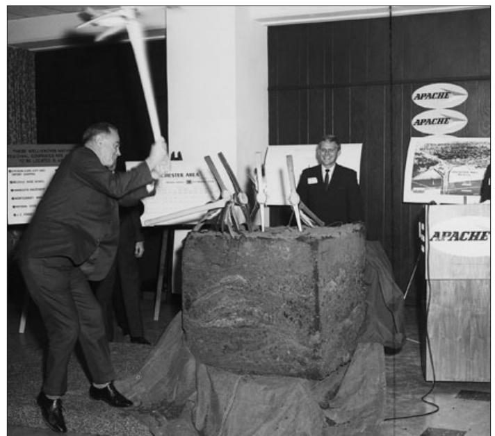
The block of frozen earth was symbolic, but Raymond Plank's heave of a pickaxe was genuine enough at the groundbreaking ceremony for the Apache Mall Shopping Center on a frigid winter day in Rochester, Minnesota.
