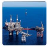
The Beryl Alpha platform is a fixed condeep gravity based structure (GBS) located in Block 9/13a in the UK sector of the North Sea - approximately 335 km north east of Aberdeen. It is located some 8 kilometers south of the Beryl Bravo platform at a water depth of 117.5 metres.
